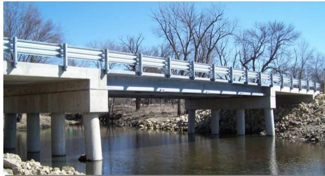
Figure 15. Photo. Jakway Park Bridge, Buchanan County, IA
