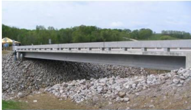
Figure 13. Photo. Mars Hill Bridge, Wapello County, IA
